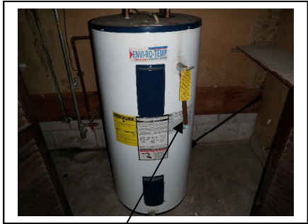
Aged Hot water heater , No Pan , and TPR extension pipe is not correct
