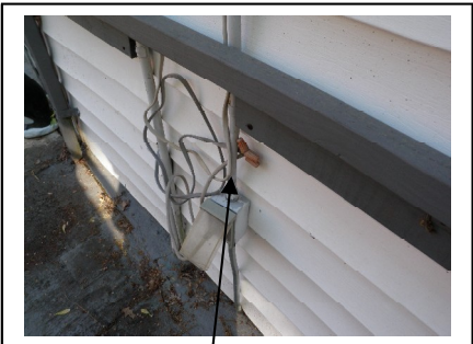
Splice wires at left side of detached garage
