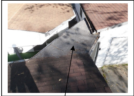
Damage Flat roof and damage to gutters
