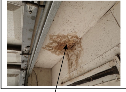
Moisture Stains in side Detached garage
