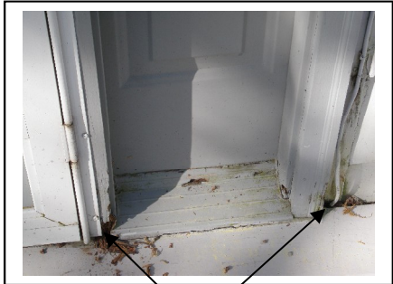
Moisture damage to trim around front door
