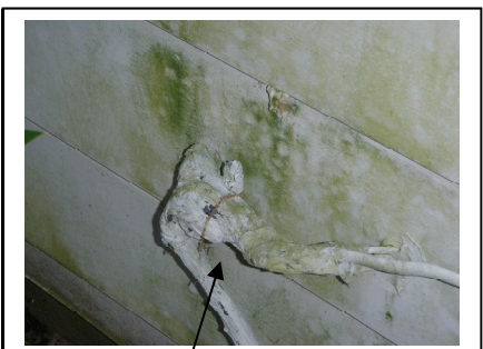
Spliced nwires/at left side of home
