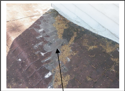
Damage valley on roof that has at some time leaked to sun room
