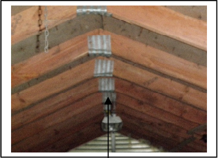
Various Trusses Damage and chords are missing in attic
