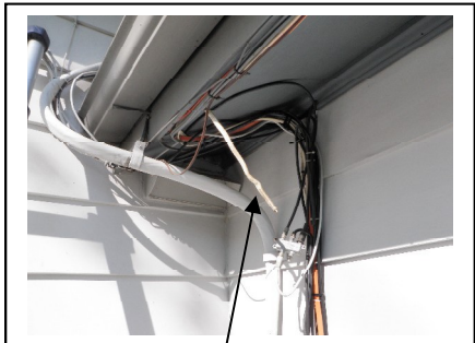
Loose Electrical wire at right side of sun room
