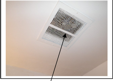
Noisy bath fan at master bathroom
