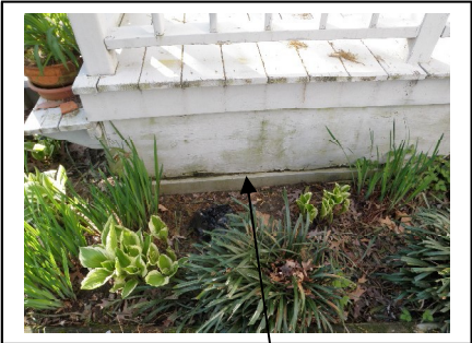
Moisture damage to skirting around rear porch
