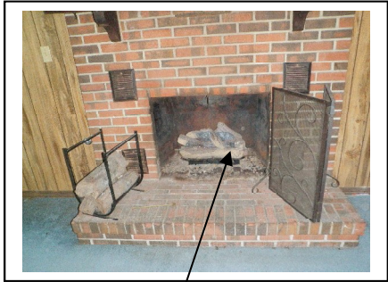
Gas log fire place / not tested ((Recommend a license chimney sweep inspect and service )
