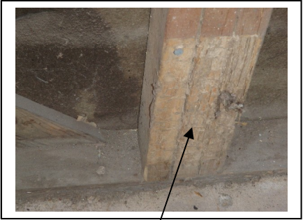
Termite Damage to Structure members in detached Garage
