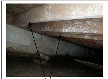
Various Termite damage to Floor framing in crawl space at front of home
