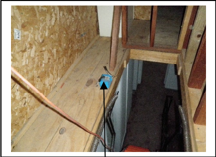
Open electrical box in attic
