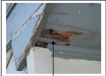
Moisture damage to Exterior trim and soffit at home and detached garage and other buildings
