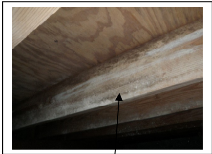
Mold and fungus like formations on subflooring in crawl space
