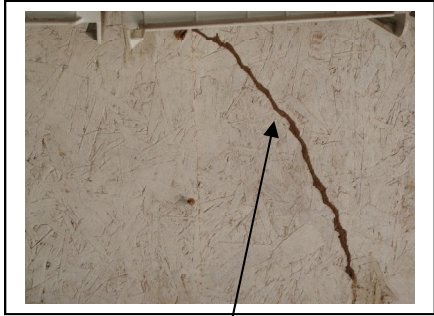
Termite Tubes In Detached garage
