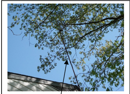
Loose Old TV Antenna at ridge of roof
