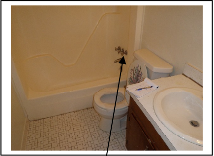
Plumbing fixtures that do work , hard to turn
