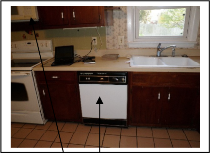
Dishwasher loose at counter top and aged Microwave
