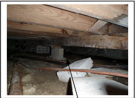
Temporary columns under kitchen area in Crawl space
