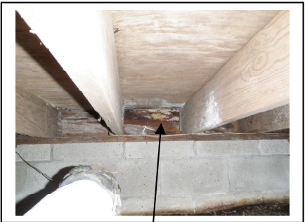
Moisture damage to rear Band board and sill plate at rear door under porch in crawl space
